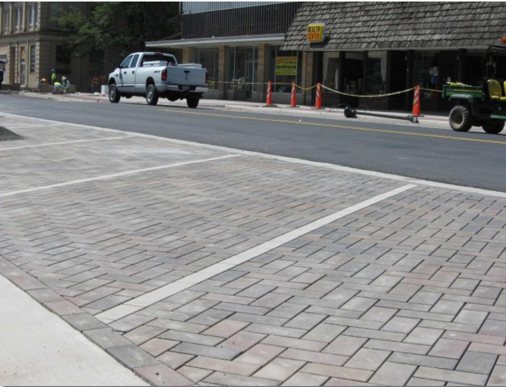
FIGURE 9.5 – EXAMPLE OF USING PERMEABLE PAVEMENT FOR PARKING SPACES IN A PUBLIC STREET PROJECT
