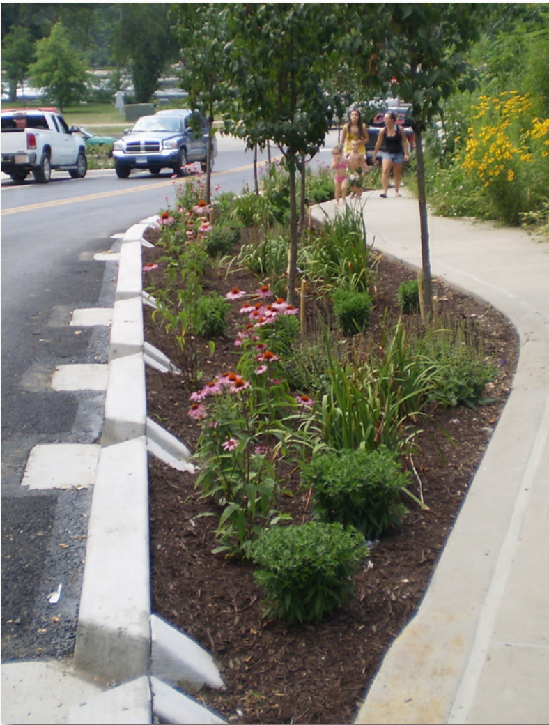
FIGURE 9.2 – STRUCTURAL BMP – DEPRESSED PLANTER COLLECTING STORMWATER FROM THE STREET
